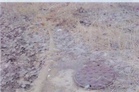
Date: 2/27/09 Photo by: CK Comments: Signs of Overflow was evident at the upstream manhole where a diversion trough was built.
